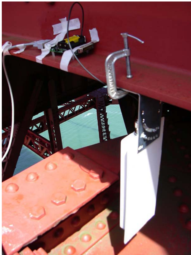
Figure 2.18: Antenna Installation on the Golden Gate Bridge
