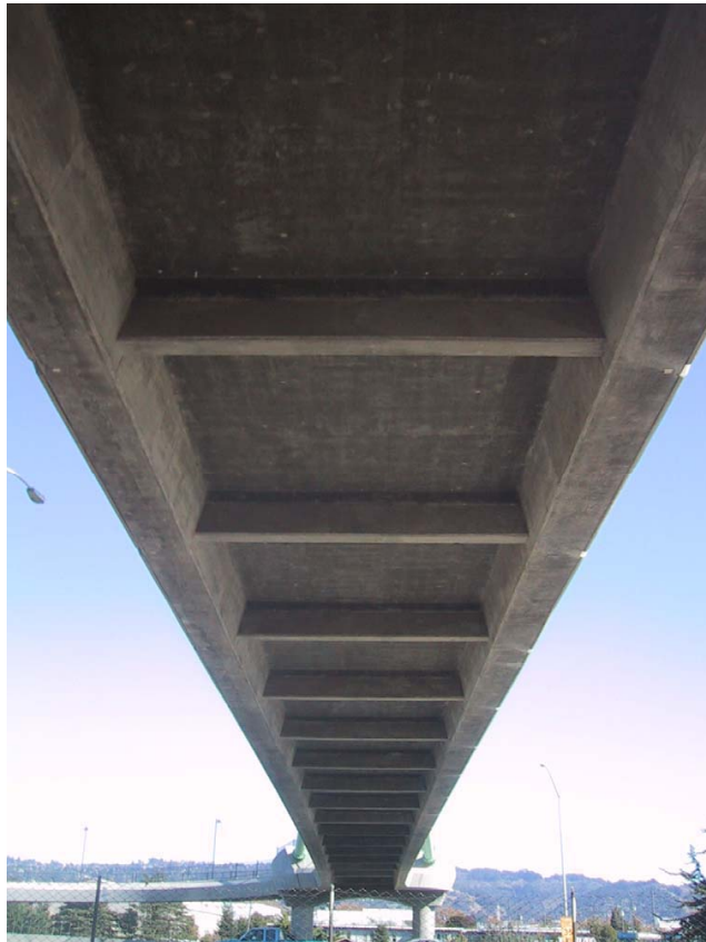
Figure 5.10: Beams Supporting Span
